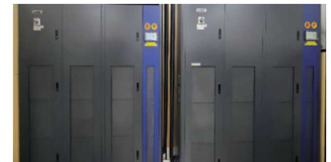
HVAC Upgrade: Replacing 20RT with 30RT Units
